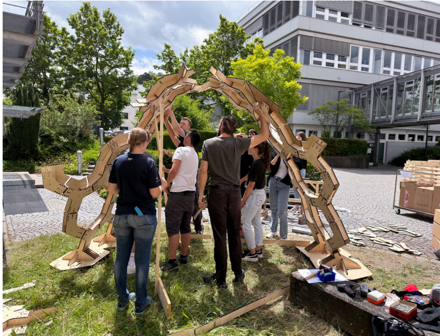
Arch closure between A and C
