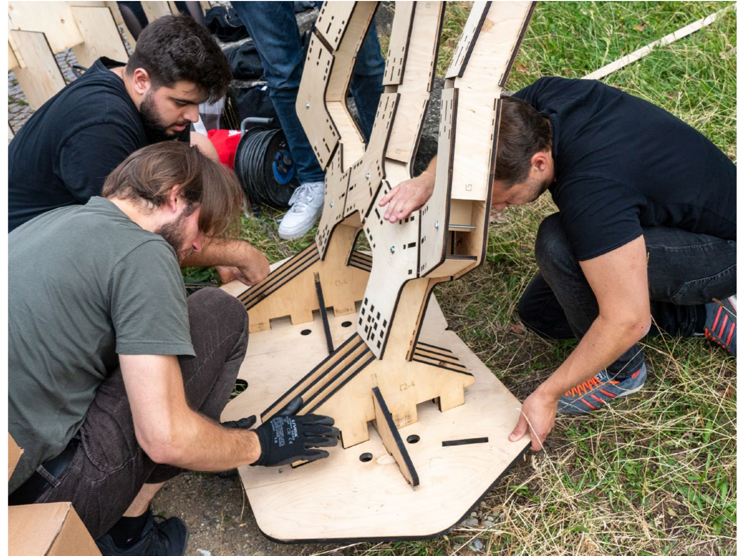
Assembling the pre-assembled Segment C onto the corresponding support plate
